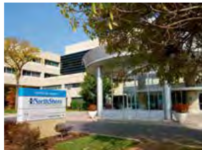
NorthShore Glenbrook Hospital
