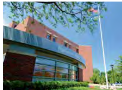
NorthShore Highland Park Hospital
